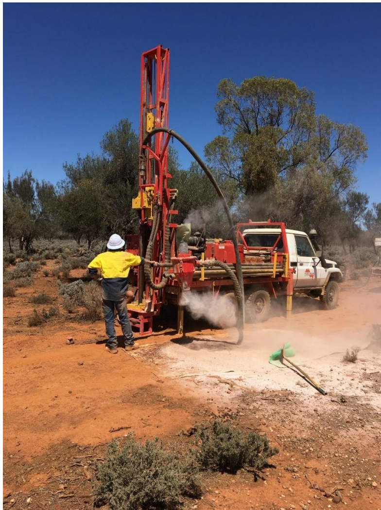
Image 2. Drill rig on site at Franklyn Project.
